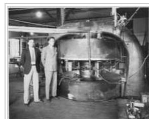
M. Stanley Livingston and Ernest O. Lawrence ( right ) in front of Lawrence's 27 inch cyclotron at the Lawrence
