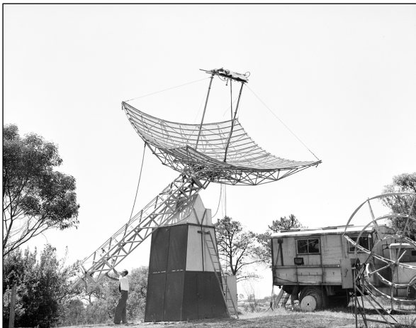
Figure 4: The 16-ft x 18-ft paraboloid at Potts Hill (courtesy: ATNF Historical Photograph Archive).
